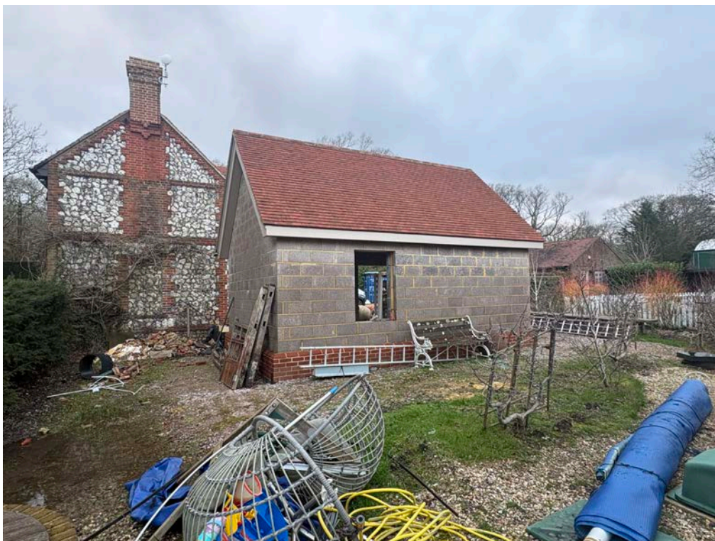
This photograph illustrates the existing garden room, still under construction. The small additional extension to be built onto this East elevation.
