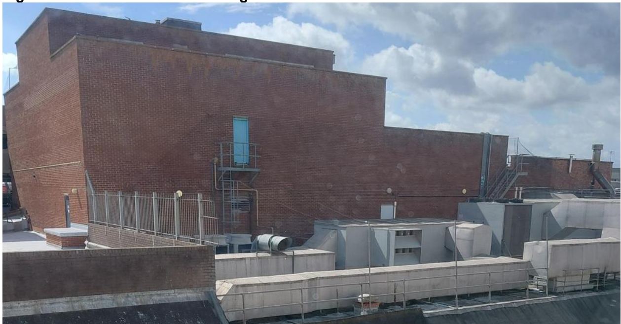
Figure 5.1: Plant at Rear of Building
