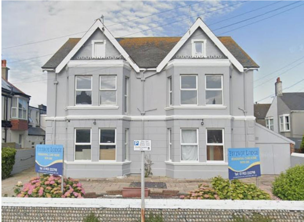
Fitzroy Lodge viewed from Windsor Road
