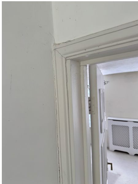
Existing non-original architrave to front bedroom
