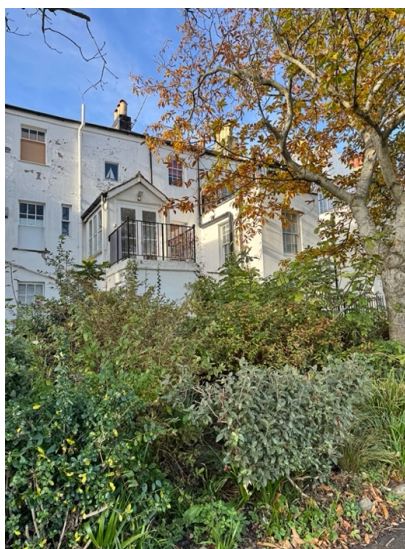
View of neighbours rear extension and second floor flat room beside
