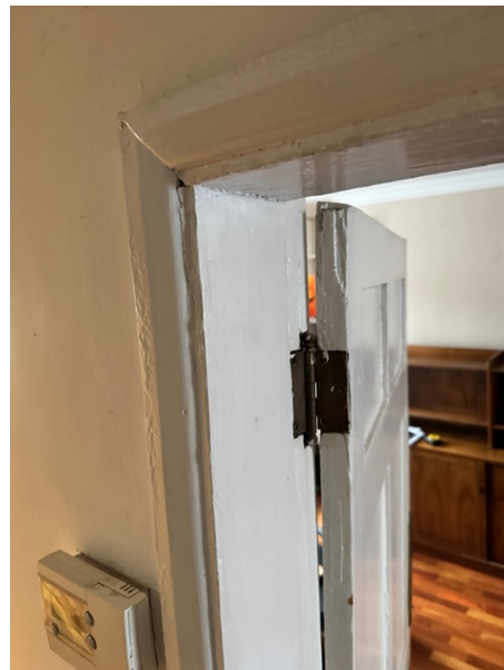
Existing non-original architraves
