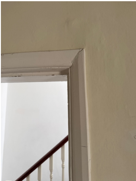
Existing non-original architrave to rear bedroom
