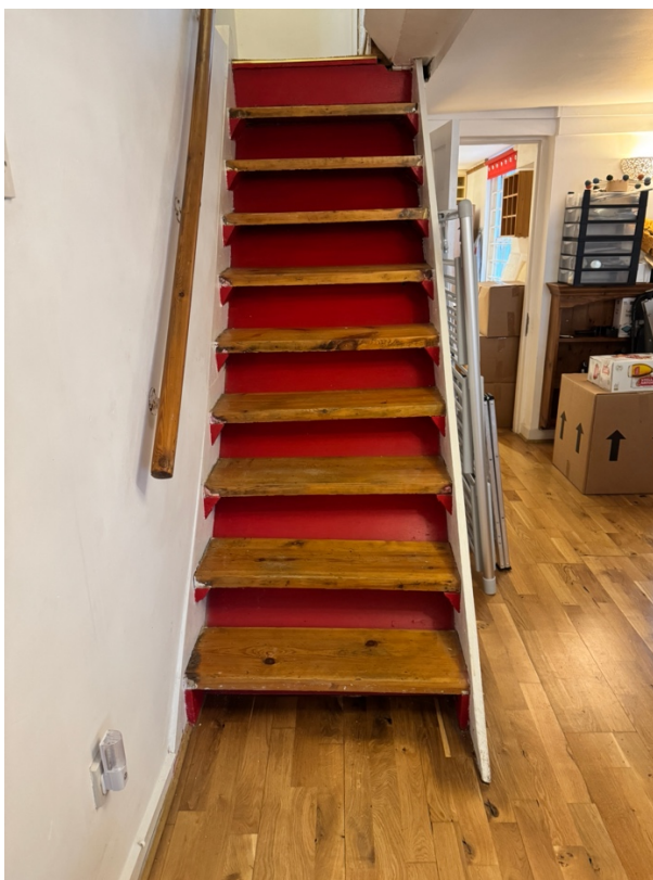
Existing staircase which is not original
