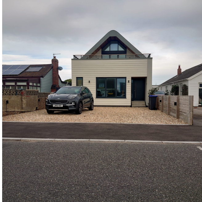
Example 3: Old Fort Road, Shoreham Beach
