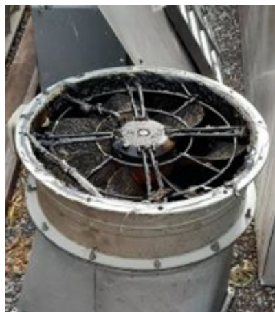
kitchen window which is completely rotten and loose, commercial extractor vent in very poor state and broken.
